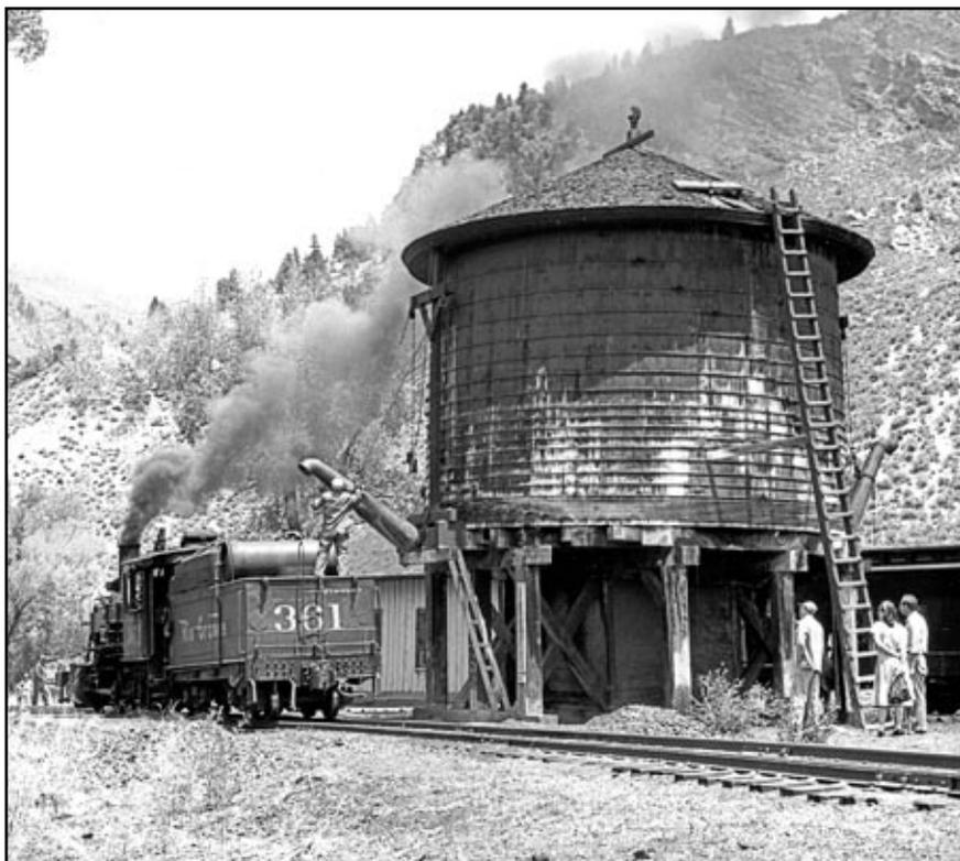
D&RGW engine 361, a 2-8-0, originally Crystal River RR No. 102, Baldwin 1900, acquired by the D&RG in 1916. These locomotives sometimes were referred to as “Little Mudhens.” This engine was dismantled at Pueblo on November 15, 1951. This scene is at Cimarron taking water prior to train returning to Gunnison.
