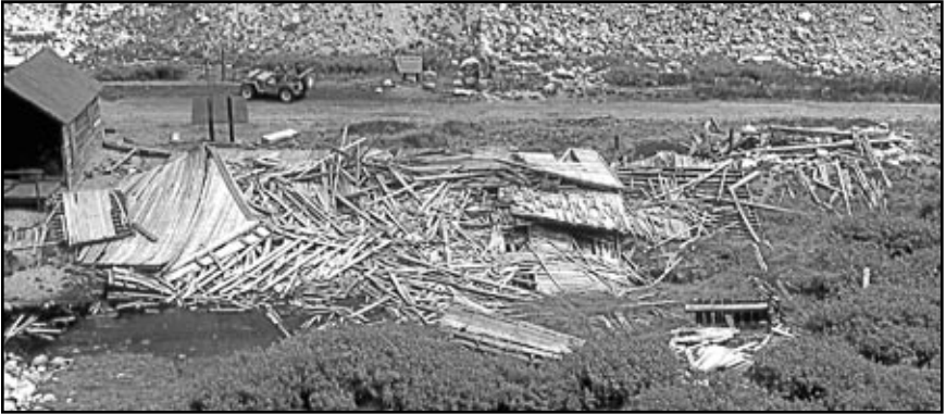
The wooden 55' x 24' boarding house was constructed 10 feet south of the depot/telegraph office. The facility housed a dining room, kitchen and two bedrooms on the lower level and a private company bedroom and large open boarding room for regular railroad crew members on the second floor. The boarding house collapsed in the early 1960s. In September 4, 1982, the wooden boarding house was a pile of lumber and building materials. – Photo © Bruce Nail.
