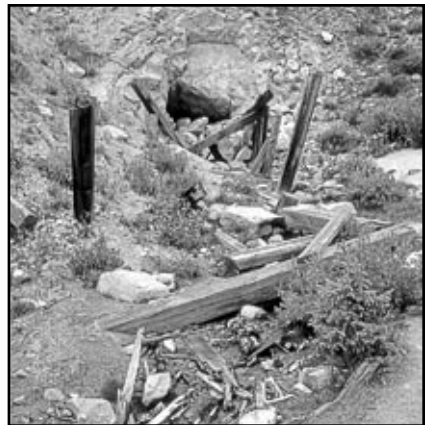
The Alpine Tunnel east portal on September 4, 1982. – Photo © Bruce Nall.
