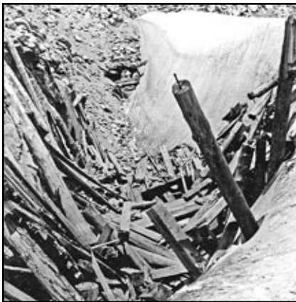
The Alpine Tunnel west portal on July 13, 1951. – Photo © Bill Abbott.
