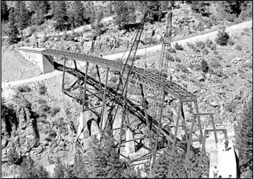
Setting the center span on the famous Devil's Gate Viaduct "high bridge." – Photo © Bill Robie.
