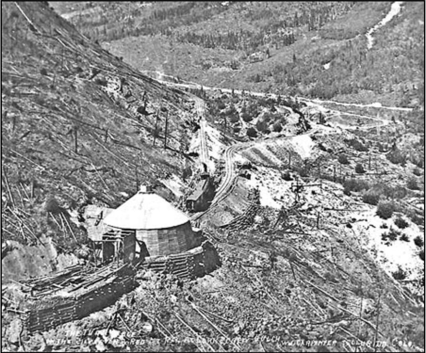
The Corkscrew Gulch covered turntable, an unusual solution on the mainline of the Silverton Railroad. – W. J. Carpenter photo.
