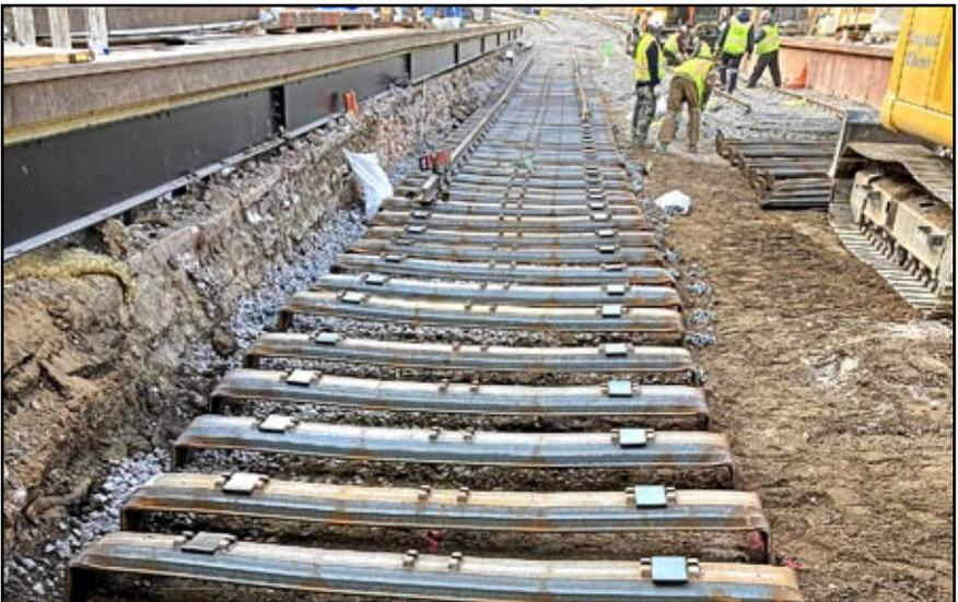
Rail installation on formed steel ties on the Manitou And Pike's Peak Railway.
