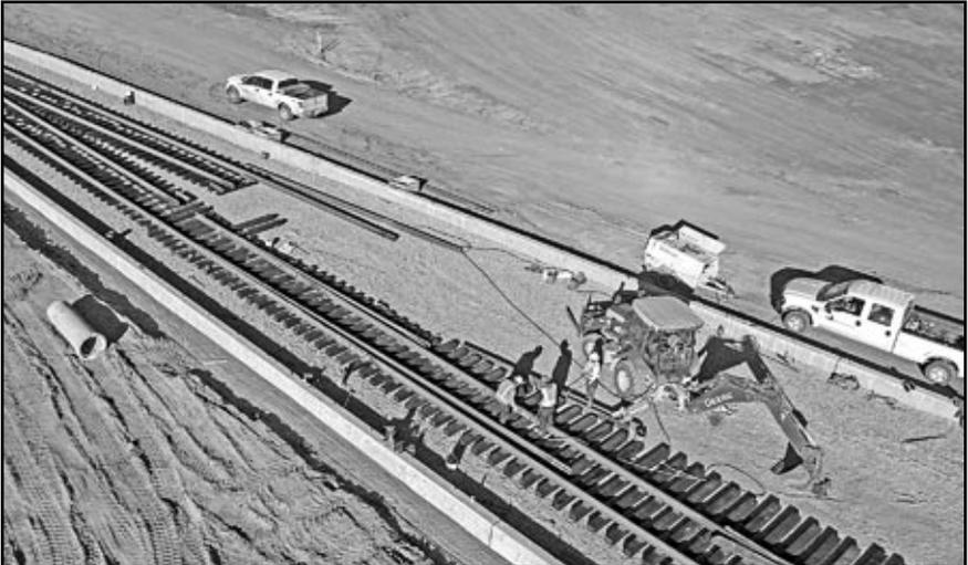
Workers installed new switches at Denver Stockyards on November 13, 2019. Denver Rock Island RR (DRIR) will shift to new trackage in 2020 and abandon the National Western Drive and Platte River tracks as part of the National Western Complex redevelopment project. The new track alignment begins at National Western Drive/Franklin Street and Race Court intersection. – Photo © 2019 by Chip.
