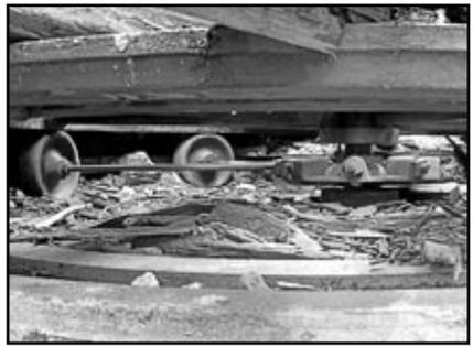
Wheels and hardware are still in place underneath the center of the turntable.
